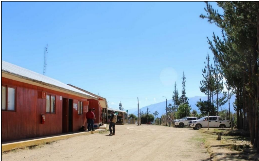
Figure 12-1: Cotabambas Base Camp
